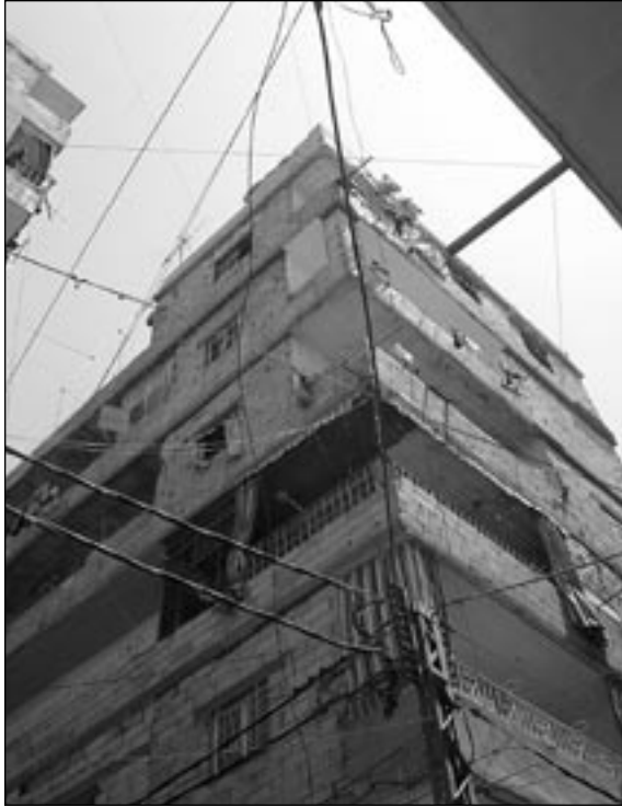
An example of the precarious and sub-standard infrastructure.
